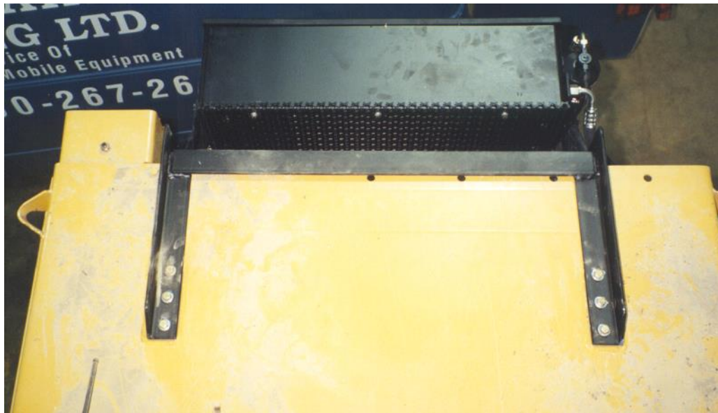
Condenser mounted with brackets in place.
